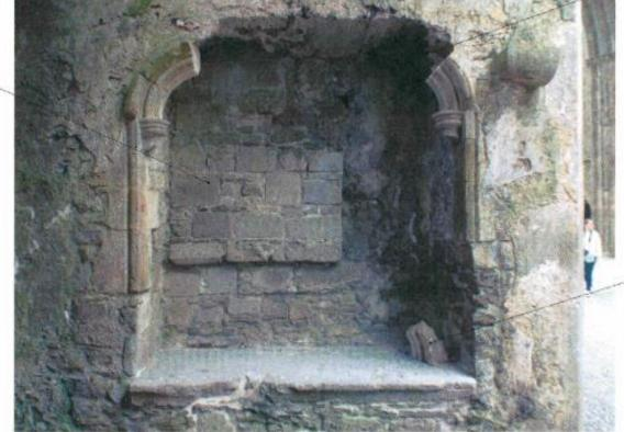
Section of stone arch that was dislodged and is to be instated
