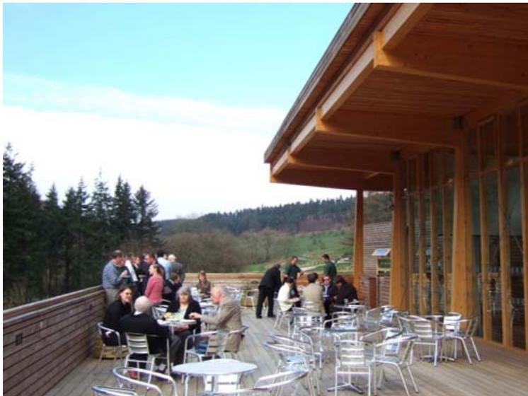
The building sits well in the landscape. It is clad in larch, grown and milled in the forest. Rainwater is harvested to flush the toilets, reducing demand on the village well. The centre is built on a timber frame and is specially designed to be recycled at the end of its life, leaving behind a minimal footprint.
